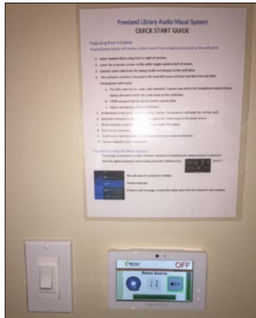
The Quick Start Guide, touch wall plate and screen lowering/raising switch is at the front of the room.
